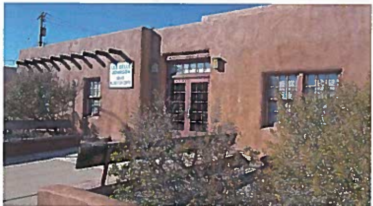
Top: Historic District commemorative plaque. Middle: Hoosier Apartments, 516 Austin Avenue, c. 1938. Bottom: Lee Belle Johnson Senior Recreation Center, 301 Foch Street, c. 1938.
