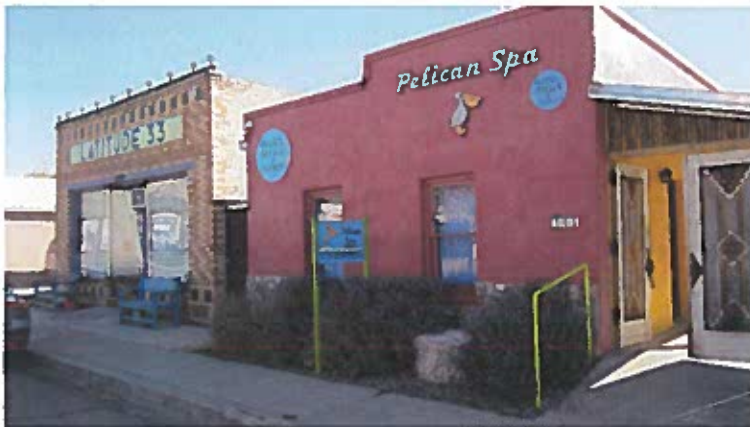
Building-mounted signs on the Pelican Spa and Latitude 33 are relatively modest in scale.
